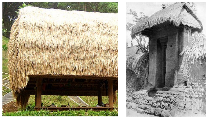
Figure 2. Examples when the alang-alang is used as roof of building
