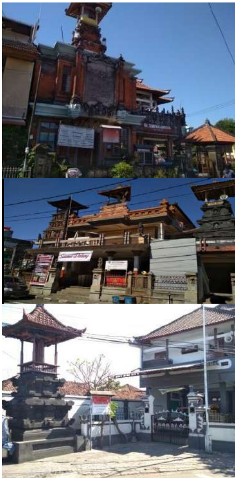
Figure 4.4 Bale banjar with two and three floors, the first floor rented is used as a fruit selling place, PAUD and kindergarten schools, bale kulkul standing on the roof plate of the building underneath, some are standing on the ground. In one area of the banjar bale building, there are three traditional banjars and at the same time three bale kulkul.
