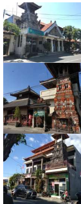
Figure 4.3 Bale banjar with two and three floors, the first floor rented is used as a savings and loan cooperative, the bale kulkul stands on the roof plate of the building underneath, there are also those standing on the ground.
